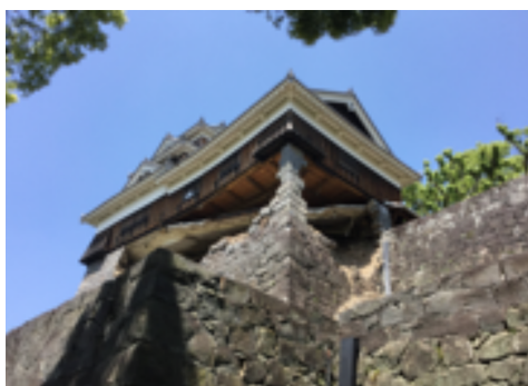
The damage of Kumamoto castle
